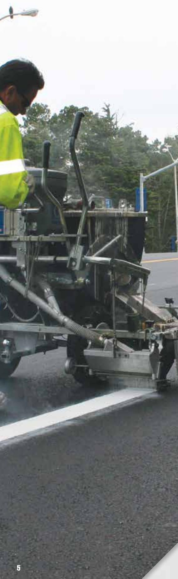
**ThermoLazer 300TC Dual PaddleMax™ System** A single chamber hopper holds 300 lb of hot thermoplastic material, reducing the need to constantly refill.
